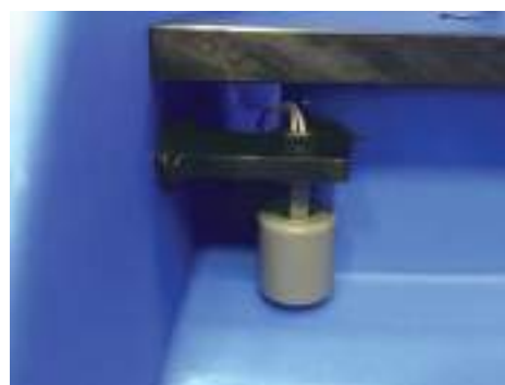
Leak Detection Sensor installed on PCS
